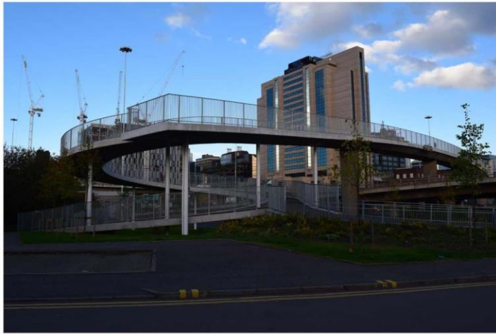
Bridge connecting Anderston to City Centre
